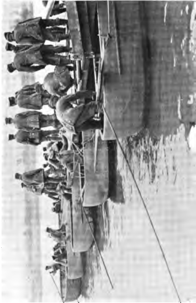
German bridge builders constructing a long pontoon bridge across the Welchael, over which their army afterward passed
